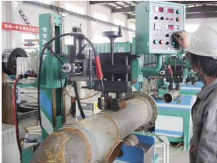
Piping Prefabrication Automatic Welding Machine(FCAW/GMAW)
