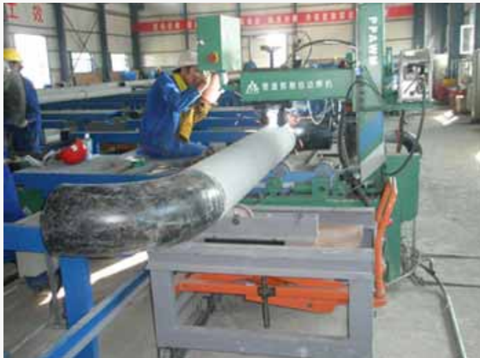
Piping Prefabrication Automatic Welding Machine(FCAW/GMAW)
